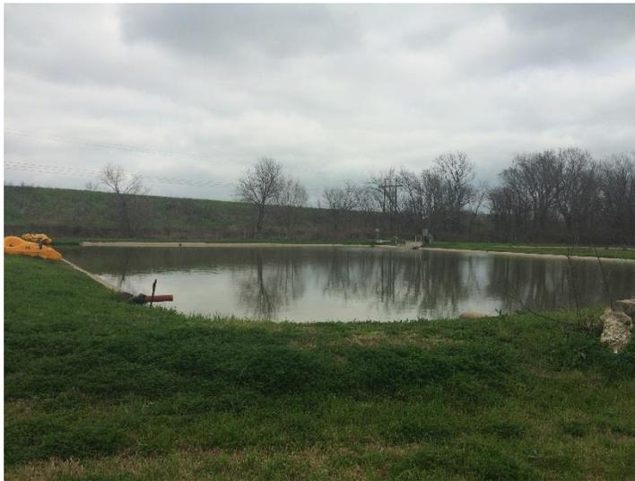
The level of water in the reclaim ponds is monitored closely by the operators as it is not monitored by the SCADA system. Water is pumped to the head of the plant or the lake when desired by the plant operators; however, flow is limited to 10% of the raw water flowrate when pumped to the head of the plant. There are currently no issues with the operation and control of the reclaim ponds.
